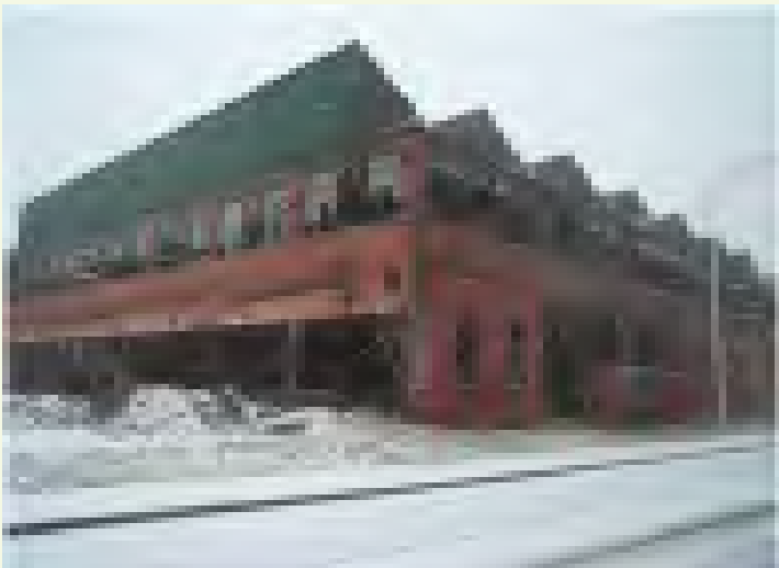
Before: Former General Cable Site
