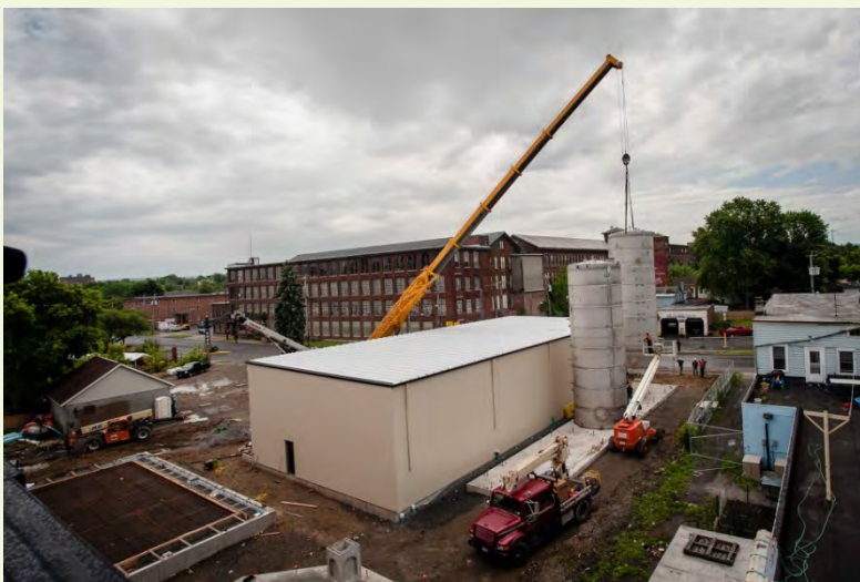
Installation of the anaerobic digester at Matt Brewing Co., Utica, NY.
