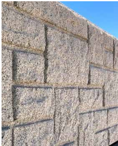
A special blend of wood shavings & cement make up this unique precast product.
