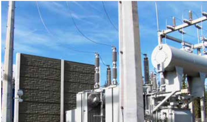
Durisol® FireStop System TORONTO, ON
