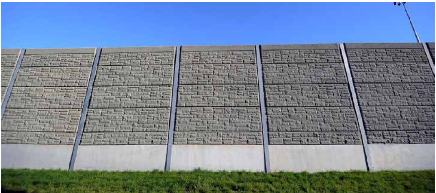
A special blend of wood shavings & cement make up this unique precast product.
