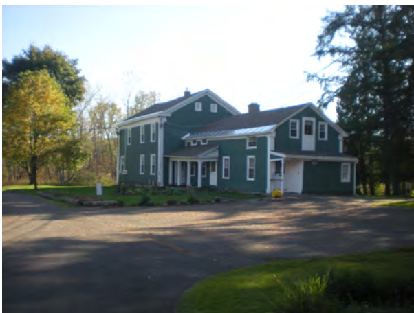
Rear of House, facing south
