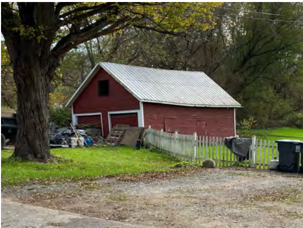
Garage, facing SE
