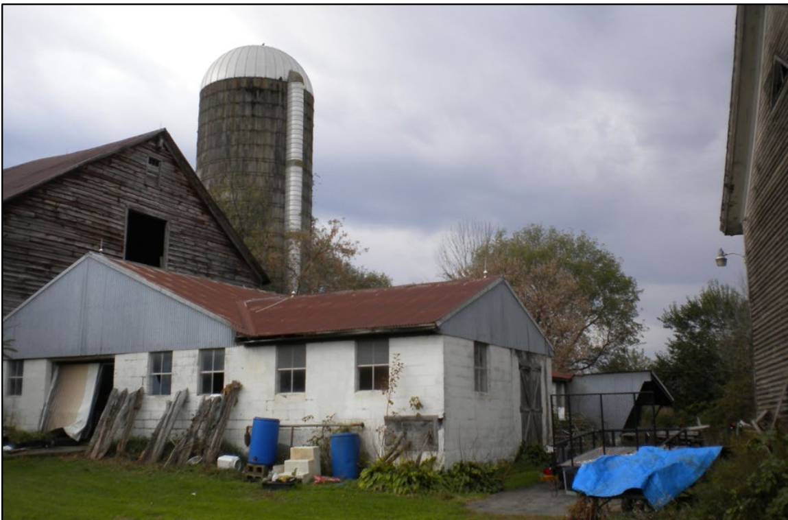
View from Auriesville Cemetery looking west toward the Project area, obscured by adjacent farm buildings.
