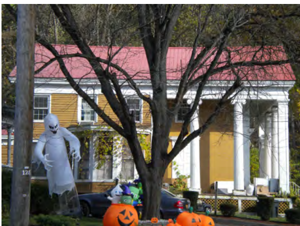
House, West Elevation, facing E
