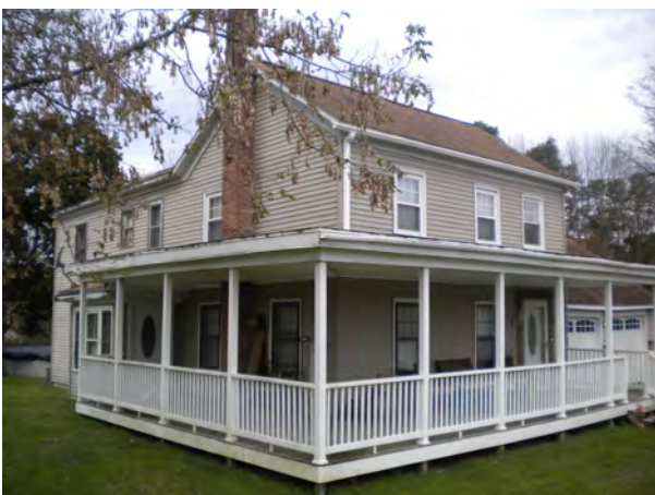
House, facing NW
