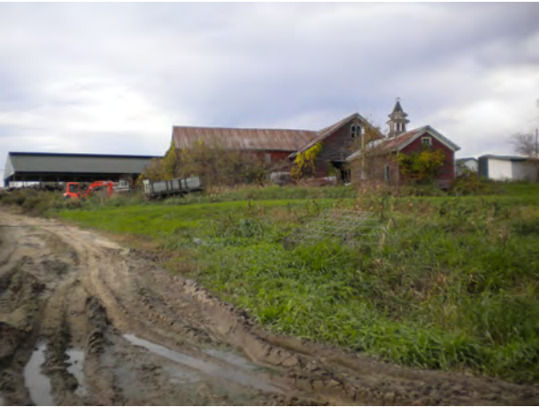
Overview of Barns, facing W
