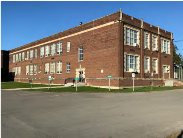
Former High School, facing NE
