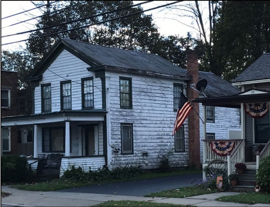
View is southwest toward the Project area showing trees in background.
