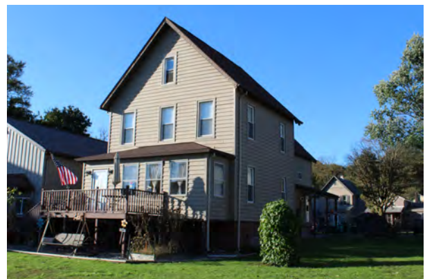
House, facing NW
