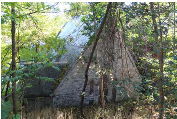
Rear Elevation, facing south
