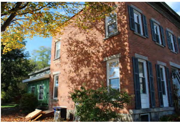
House, facing NW
