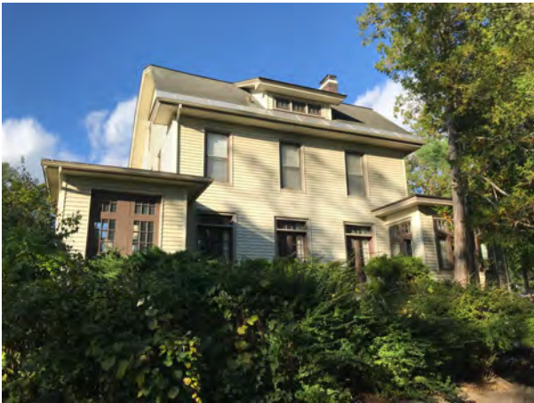
Facade, facing NNE
