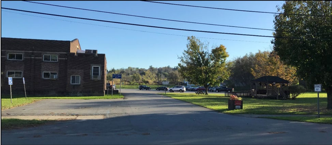
Montgomery County Public Annex; view from parking lot, facing south toward the Project area.
