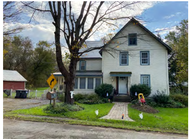
House, facing S
