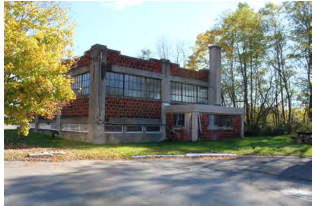
Office, facing SE
