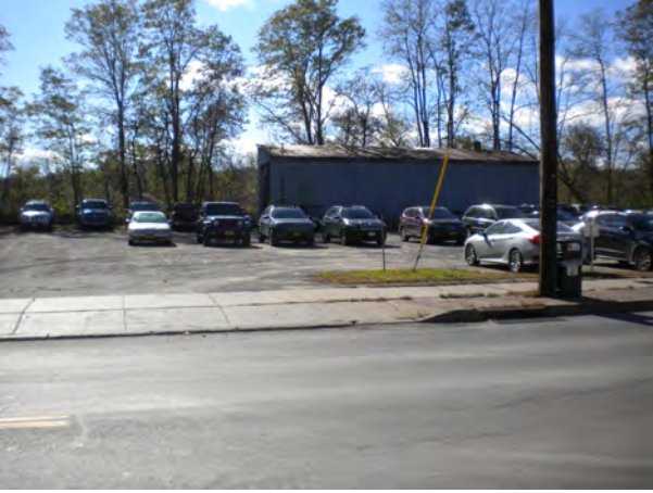
Metal Shed, facing S
