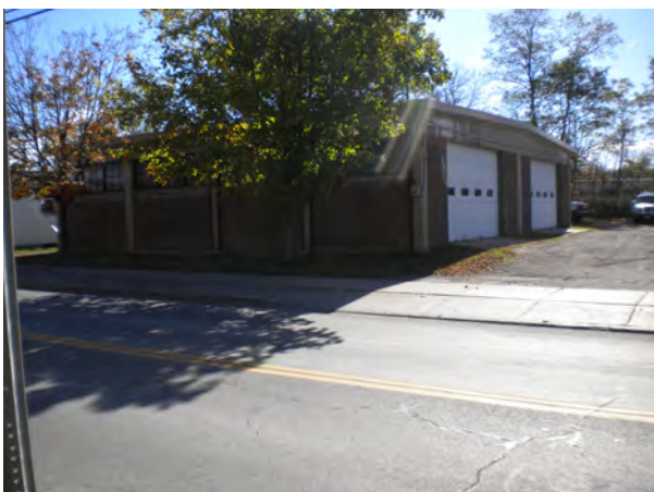
Garage facing, SE
