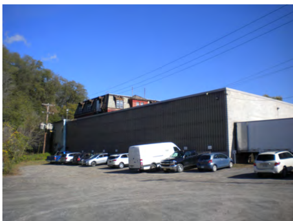
Building, facing NE
