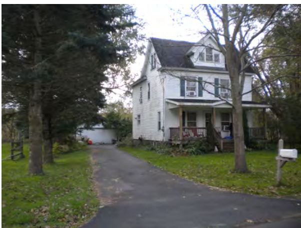
House, facing S
