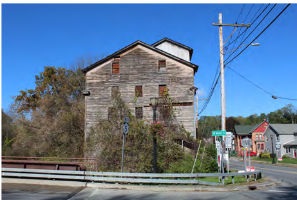
Mill, facing NW
