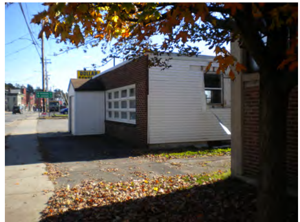
Facade, facing SE
