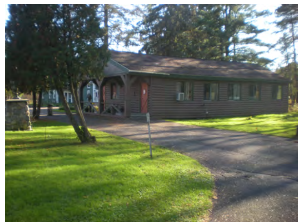
New Log Outbuilding, rear of house, facing south
