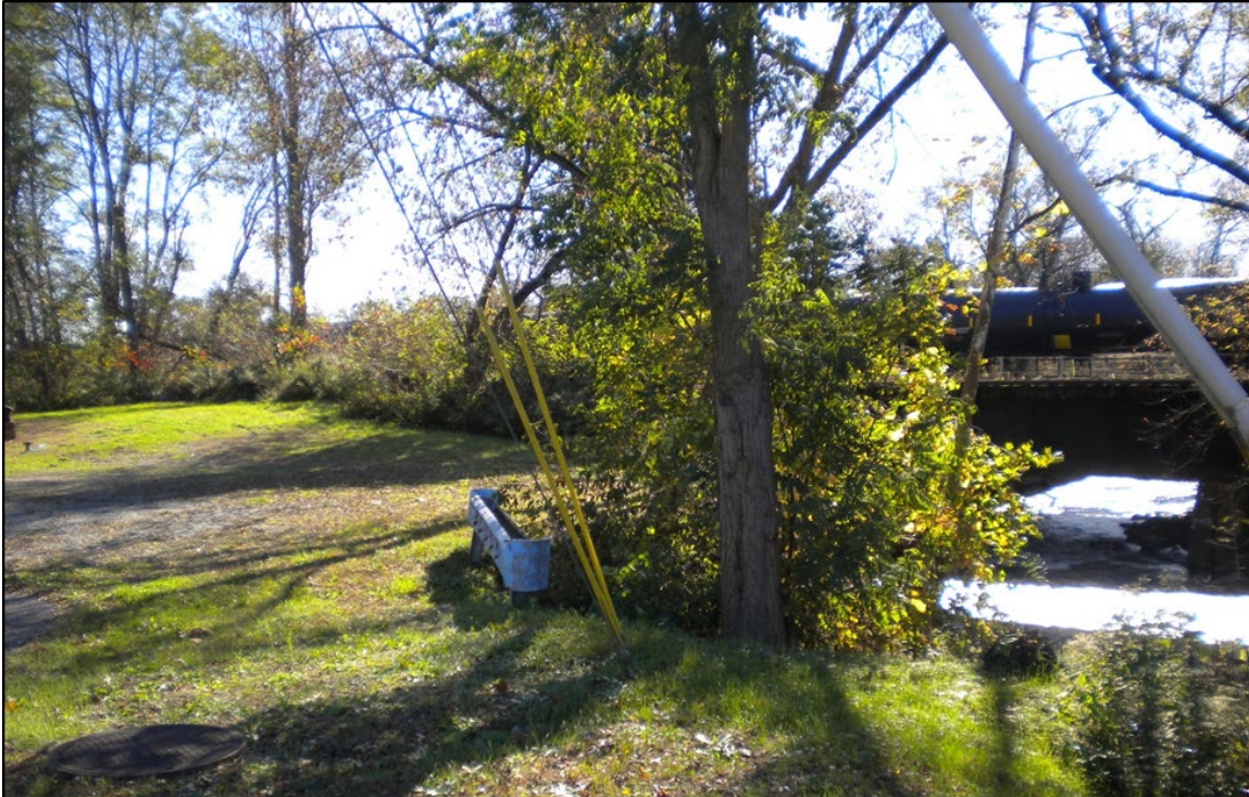
View from street at Lower Mill, facing southwest, screened by railroad and vegetation.
