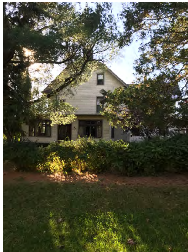
House, east elevation, facing W
