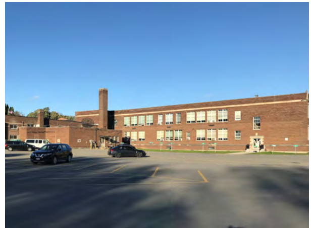
Former High School, facing NE
