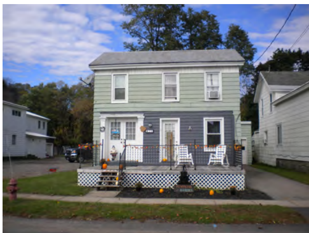
House, facing north
