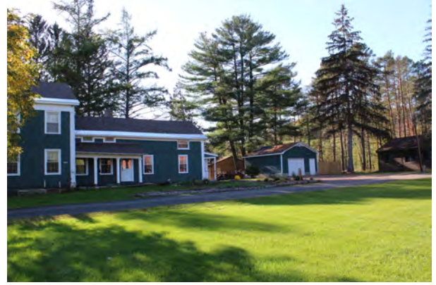
House and outbuildings, facing west
