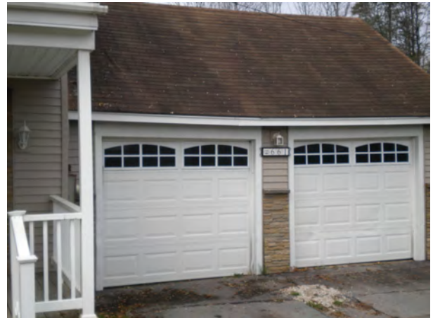
Garage, facing WNW
