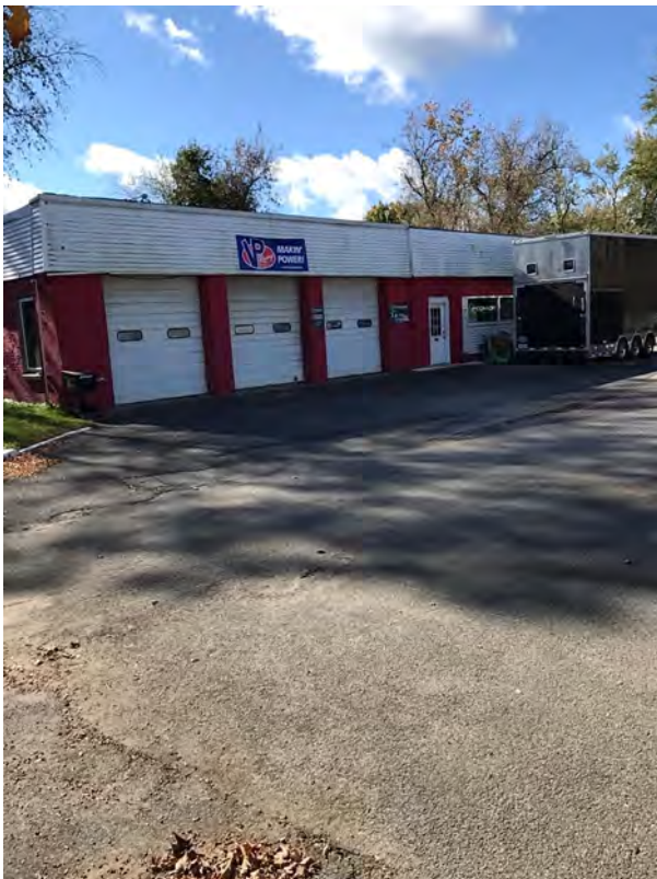
Facade, facing SW
