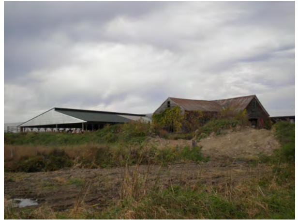
Overview of Farm, facing NW
