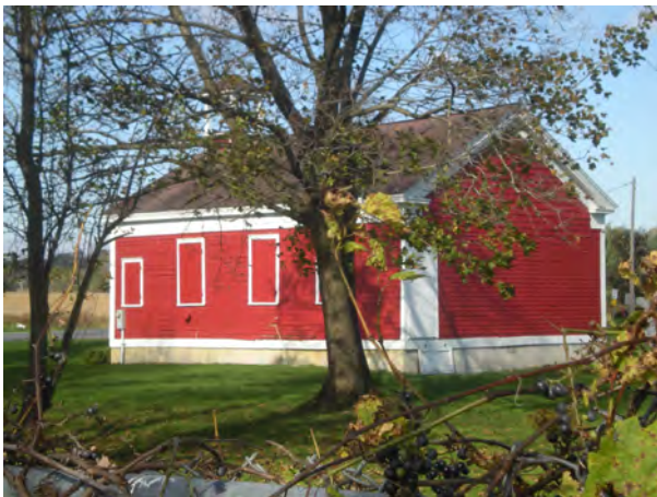
Schoolhouse, facing NW
