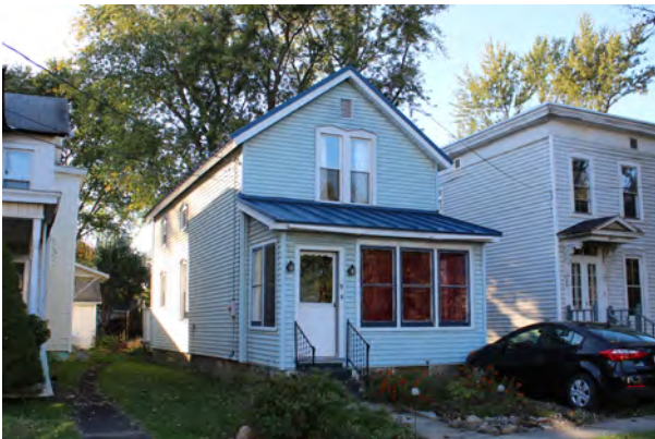
House, facing NW
