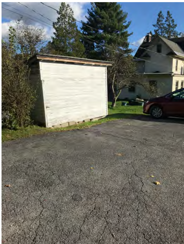
Garage, facing SE
