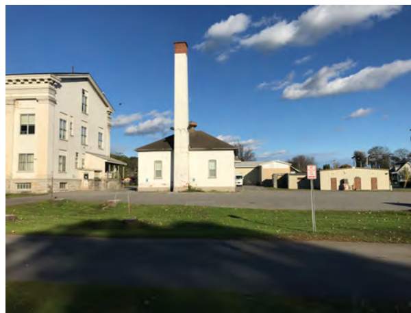
Courthouse, facing E
