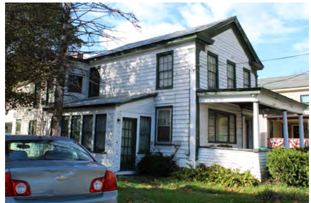
House, facing NW
