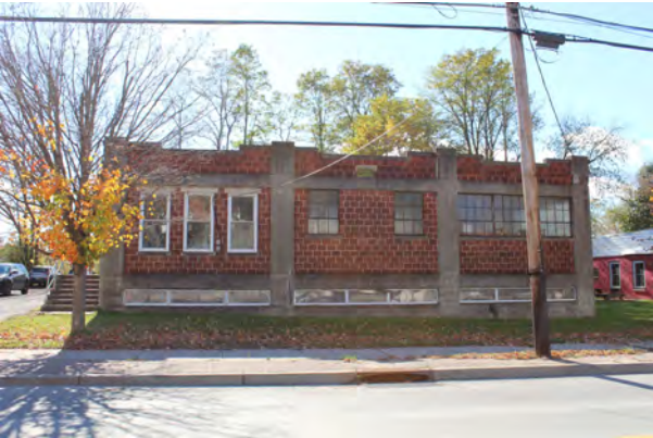
Office, facing S
