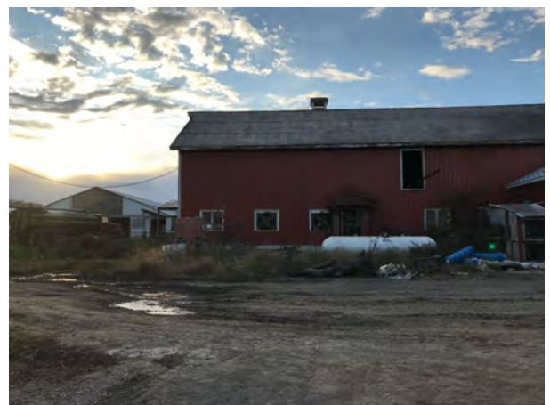
Ground Barn, facing W
