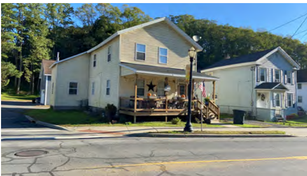
Facade (southwest elevation) and northwest elevation
