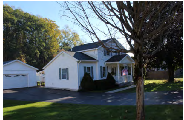
Facade and northwest elevation
