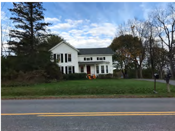
Facade, facing NNW
