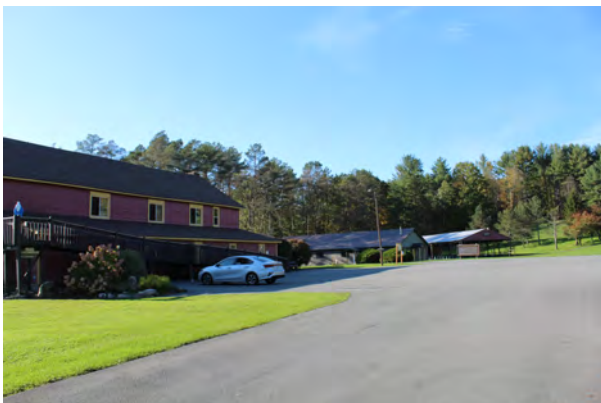
Chapel northeast elevation
