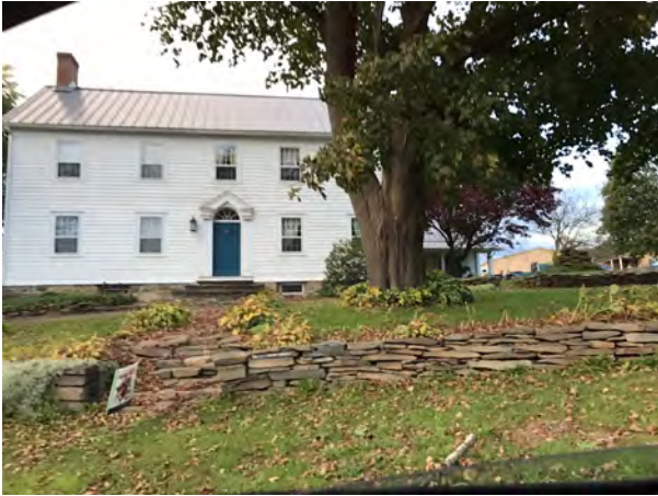
Facade, facing N
