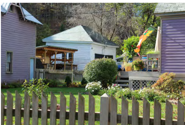
Garage, view northwest from Jansen Street
