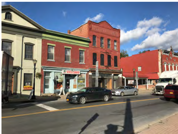
Facade, facing NE
