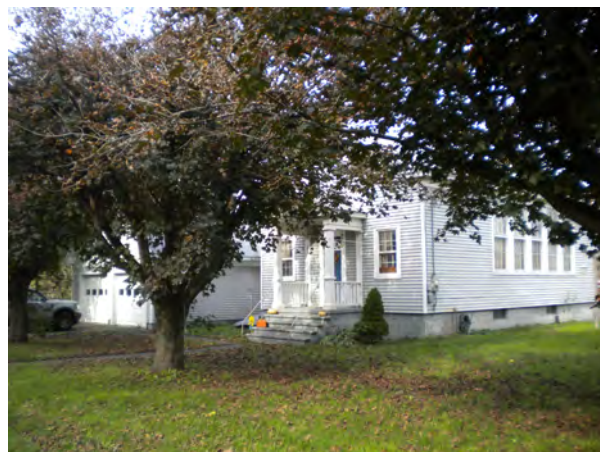
House and garage, facing NW
