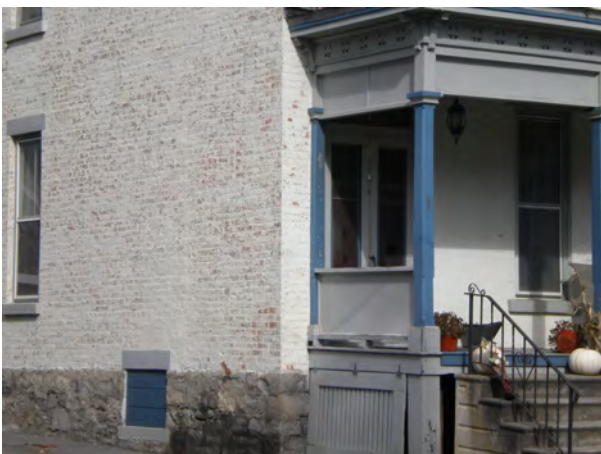
House porch detail, facing northeast
