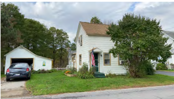
Facade and south elevation of house and garage
