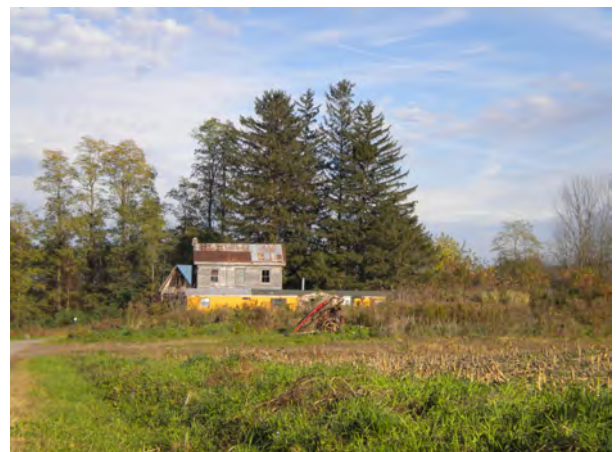
House, facing east
