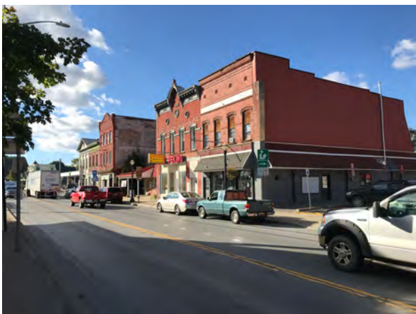
Facade, facing NW
