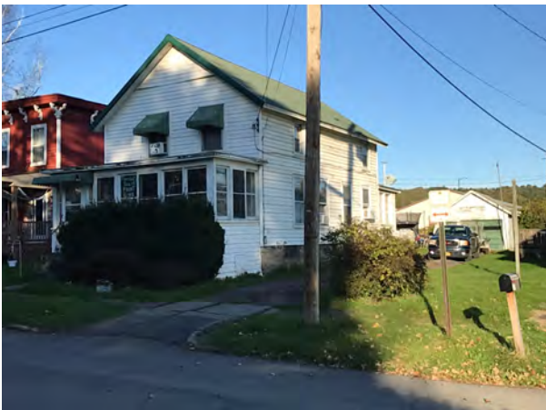
House, facing NE
