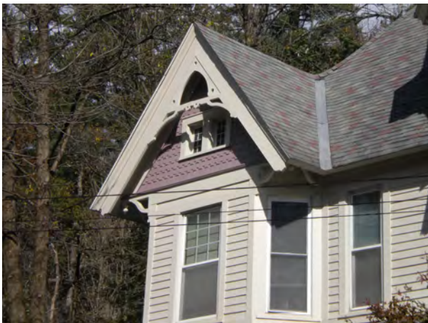
House, decorative truss work in the apex of facade gable
