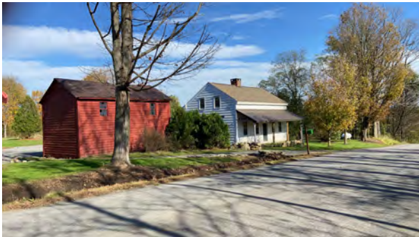
House and Barn, view northeast. Facade and northwest elevation
