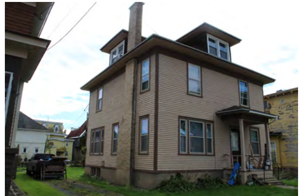
Facade and east elevation
