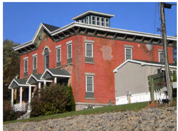
Mansion, facing NW
