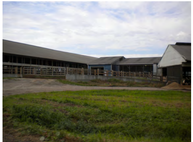
Loafing Shed, facing NW
