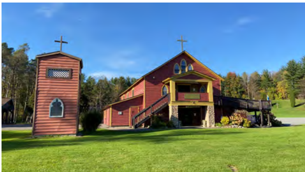
Chapel facade (southeast elevation) and southwest elevation
