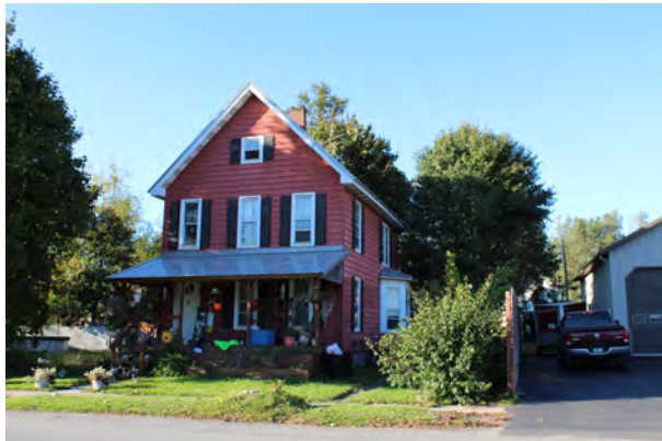
Facade and east elevation
