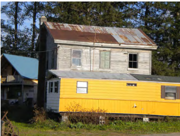
House, facing east
