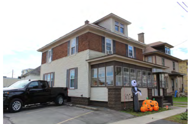
Facade and east elevation
