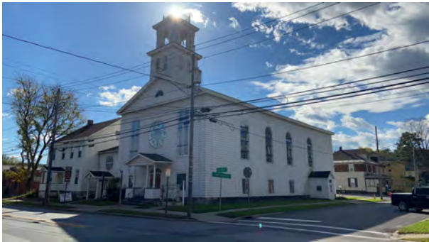
Facade (east elevation) and north elevation
