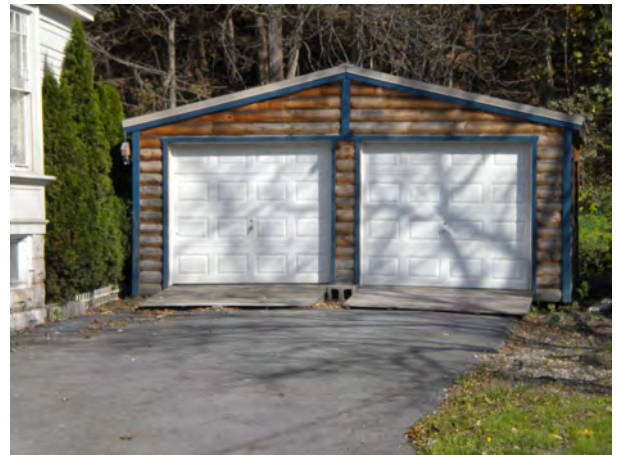
Garage, facing E
