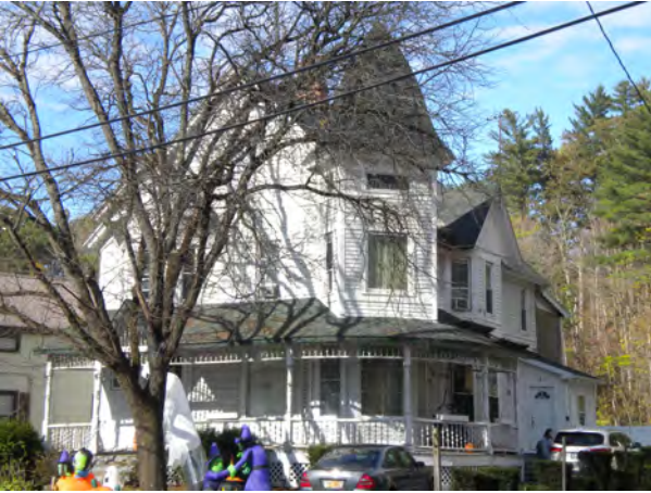
House Facade, facing N
