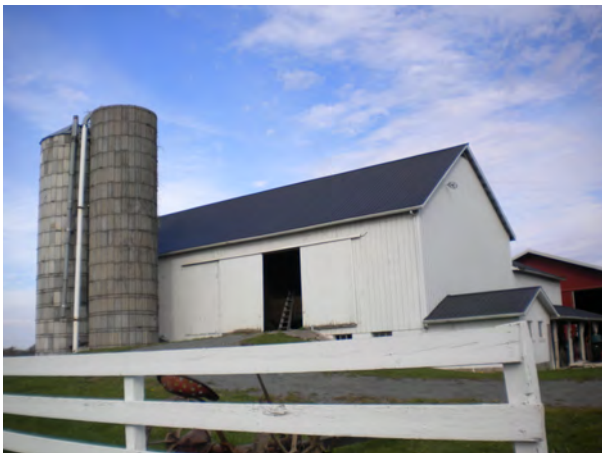
Barn and Silo, facing NNW
