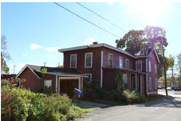
Rear, view southeast
