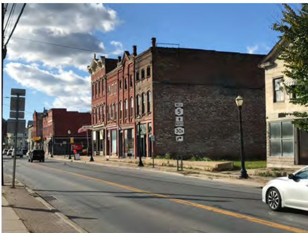
Facade, facing NW
