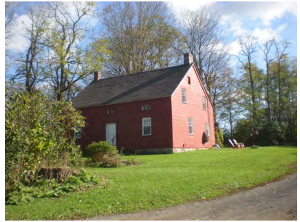
House, facing NE
