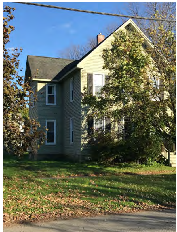
House, facing East
