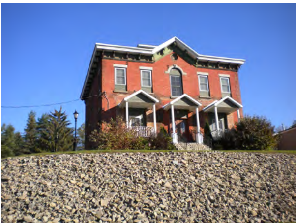
Facade, facing NNW
