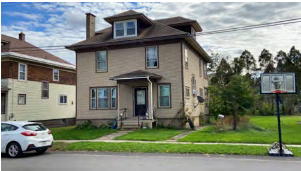
Facade (north elevation) and west elevation
