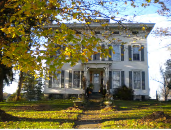
Facade, facing N
