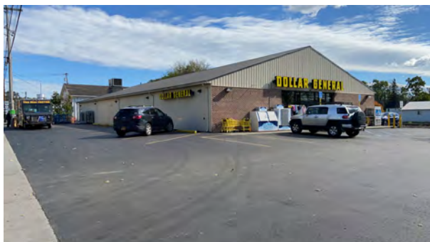
Facade (west elevation) and north elevation
