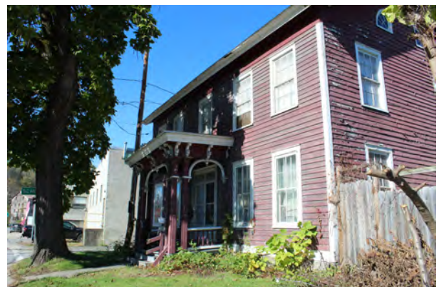
Entry porch at facade (view northwest)
