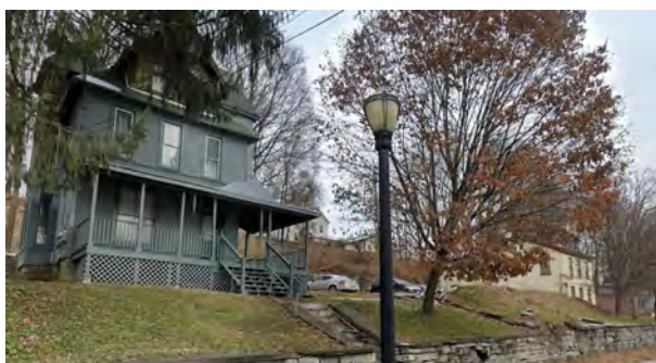
Overview, facing NE
