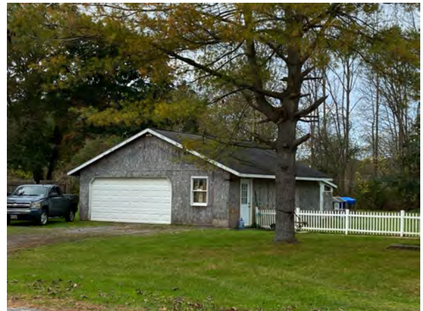
Garage, facade and north elevation
