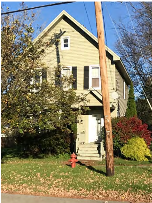
Facade, facing East
