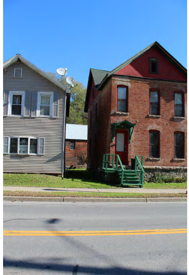
Facade and northwest elevation
