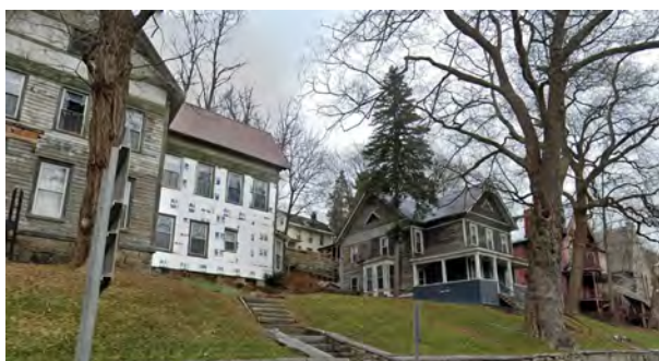
Overview, facing NE
