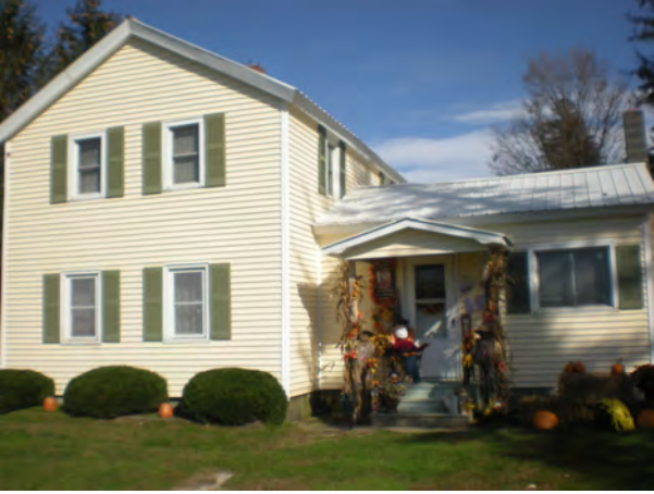
Caretakers House, facing NE
