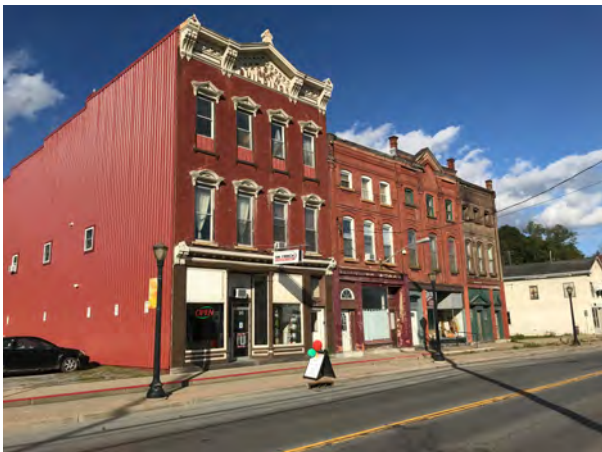
Facade, facing NE
