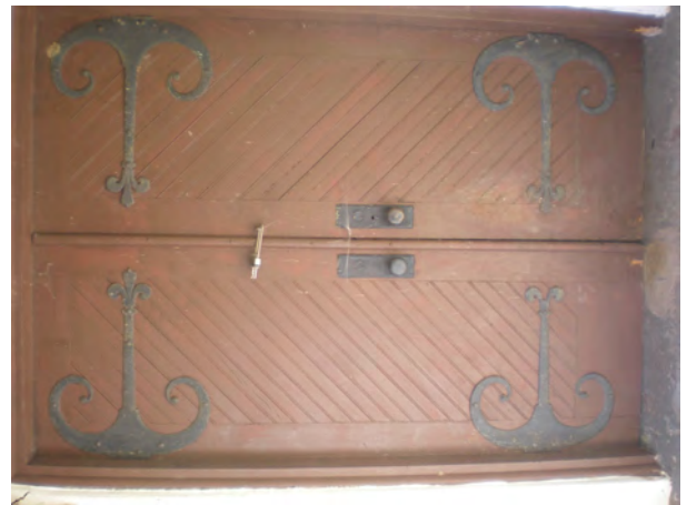
Memorial Chapel front door strap hinges, facing W
