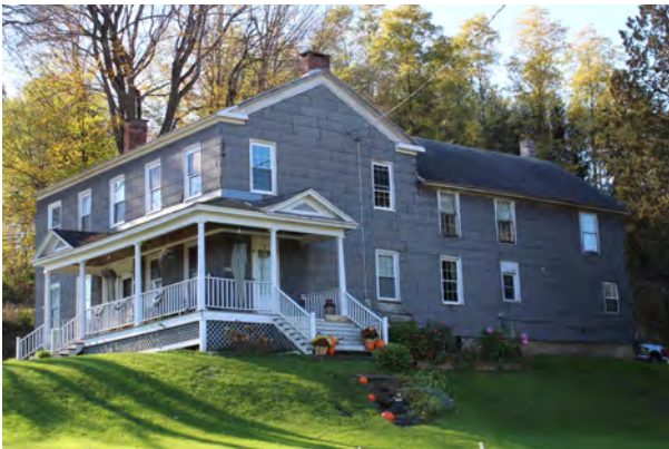
House, facing W
