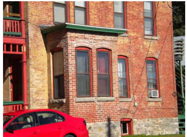
Detail of south elevation
