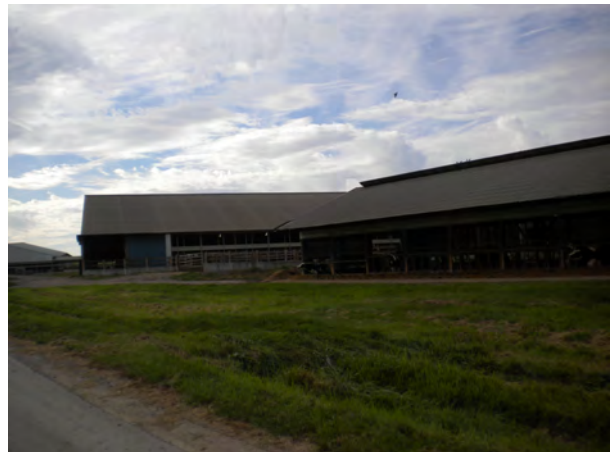
Loafing Shed, facing NW
