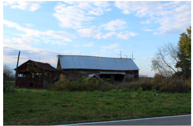
Farm Buildings, facing NW
