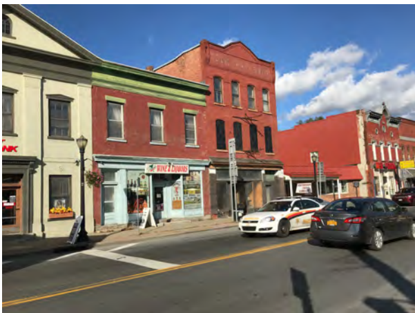
Facade, facing NE
