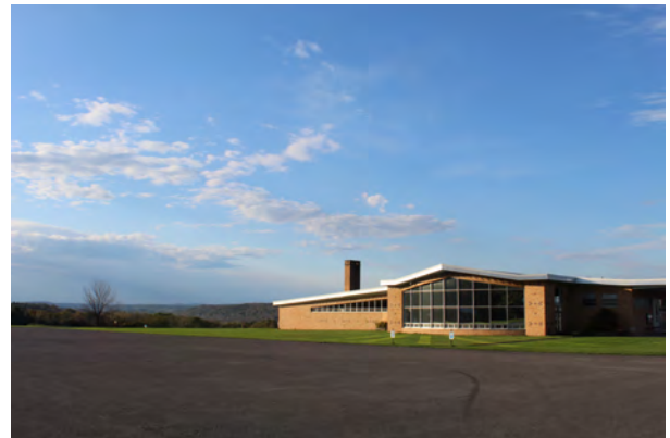
Building, facing NW
