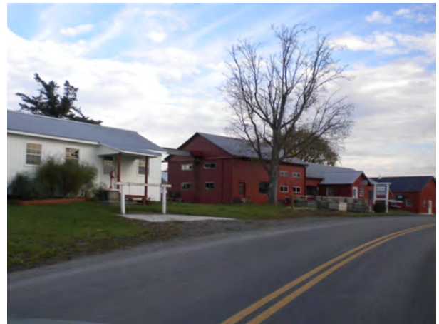
Office and Shops, facing NE
