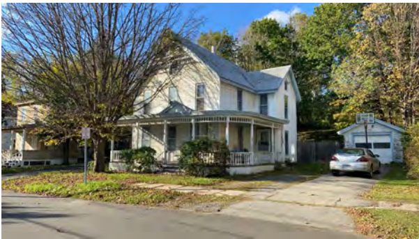
Facade (south elevation) and east elevation
