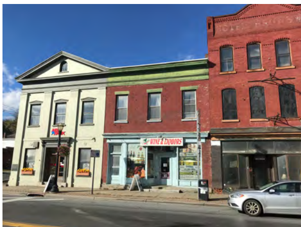
Facade, facing N
