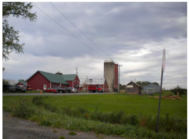
Overview of Farm Buildings at Argersinger Road and Borden Road intersection, facing NE
