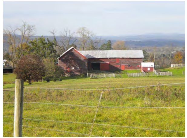
Barn and Outbuildings
