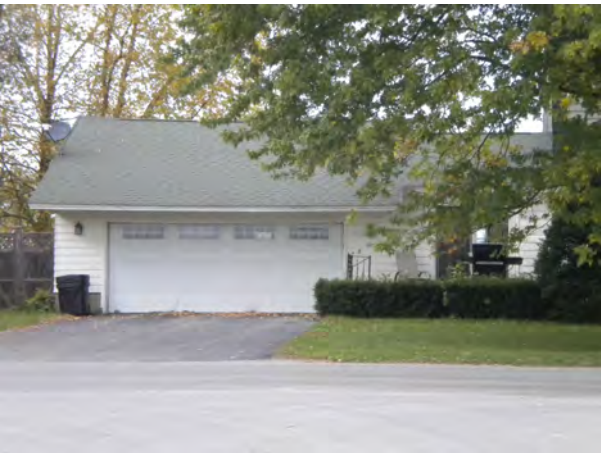
Garage attached to House, facing NW
