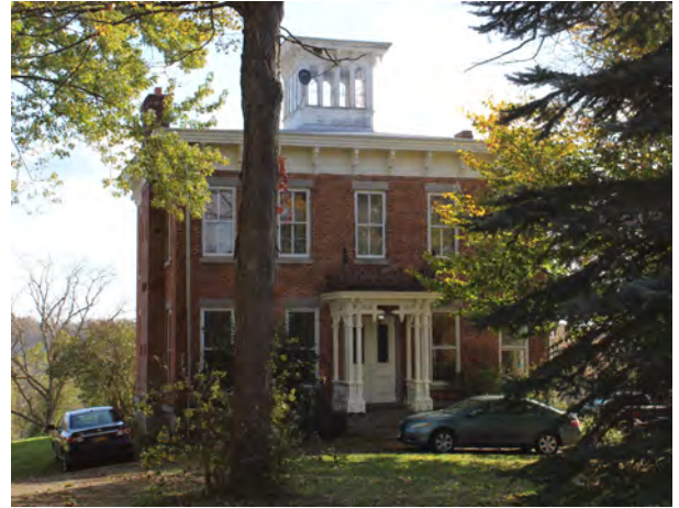
Facade, facing E
