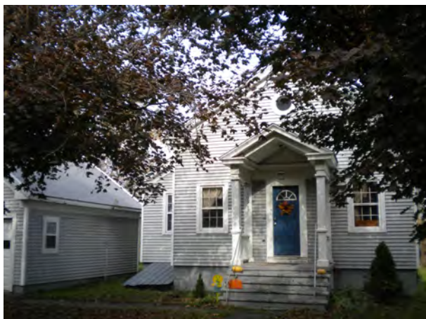
House facade, and garage, facing N
