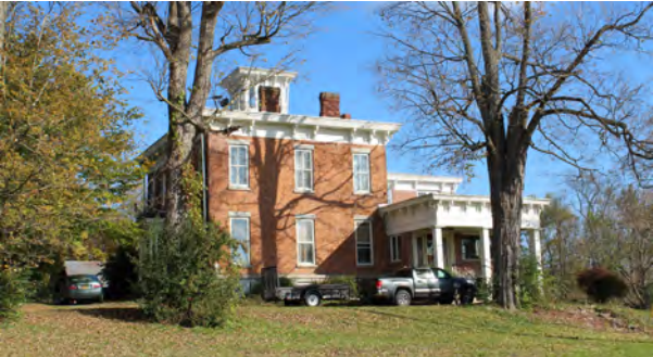
South Elevation, facing N
