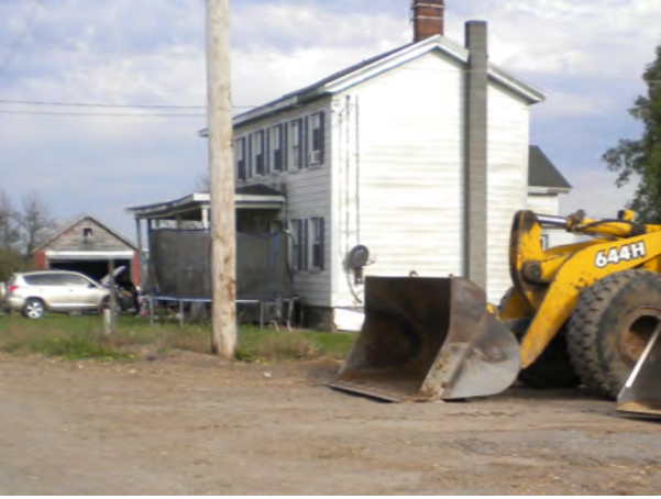
House, facing NE
