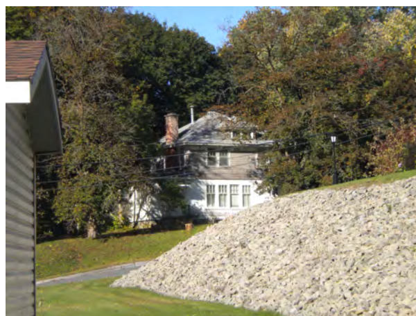
Overview, facing W
