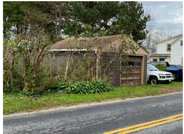
Garage, facade and south elevation
