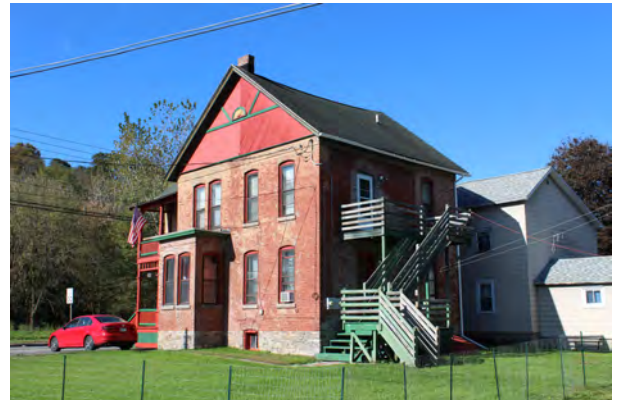
Southeast elevation and rear (northeast) elevation
