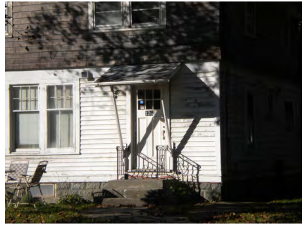
House entry, facing W
