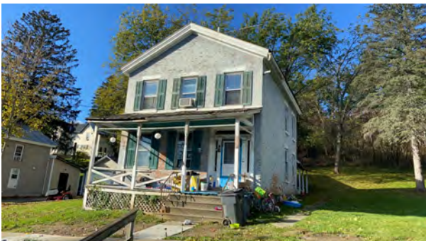
Facade (south elevation) and east elevation
