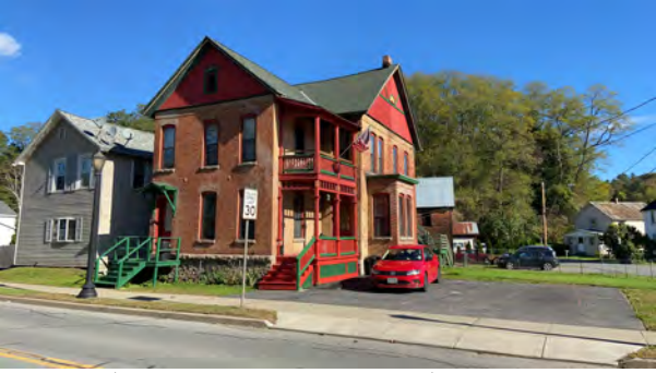
Facade (southwest elevation) and southeast elevation
