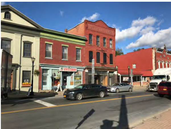
Facade, facing NE
