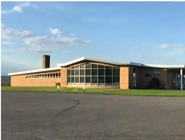
South Elevation, facing N
