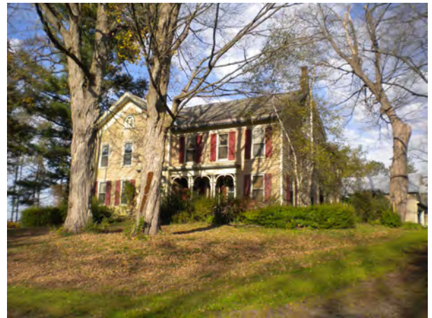
House, facing NE
