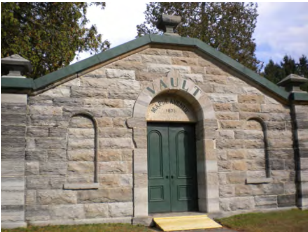
Vault, facing NE
