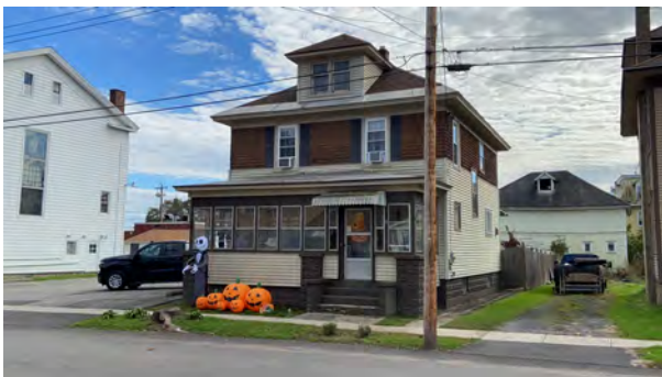
Facade (north elevation) and west elevation
