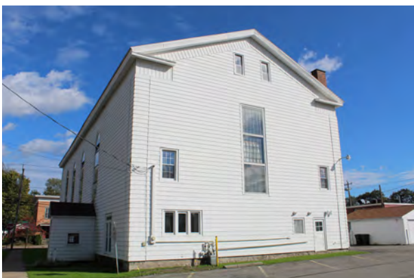
Rear (west) elevation, facing E
