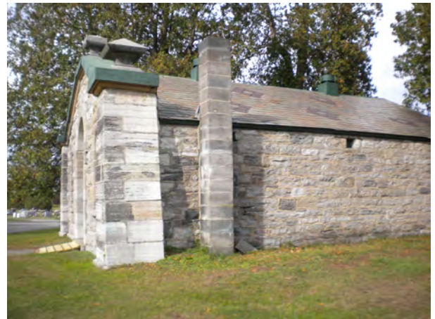
Vault, facing NNW
