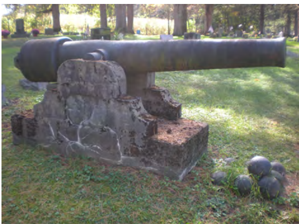
Naval Gun on concrete carriage, facing NW
