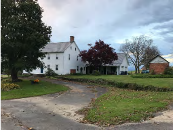
House, Addition, Smokehouse, and Driveway, facing NW
