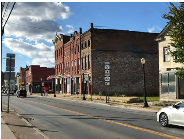
Facade, facing NW
