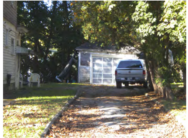
Garage, facing W
