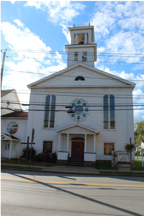
Facade, facing W
