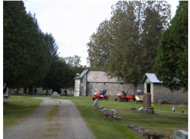
Vault and Equipment Shed, facing NW
