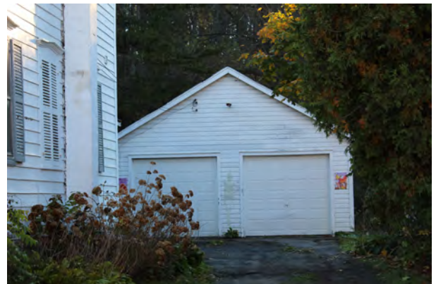
Garage, view east
