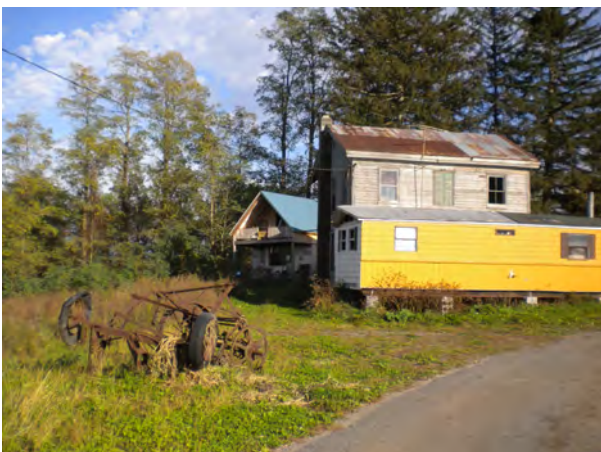
House, facing east, with addition at rear
