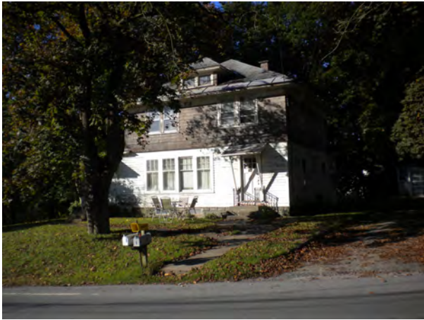
House, facade, facing W
