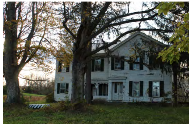
House, facing W
