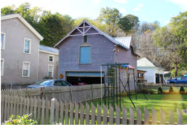
Garage facade (southeast elevation) and northeast elevation
