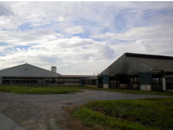
Loafing Shed, facing NW
