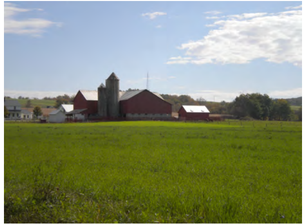
Barn, facing E
