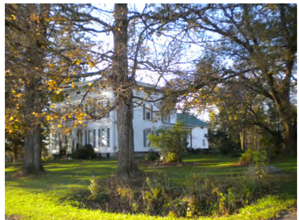
House, showing rear addition
