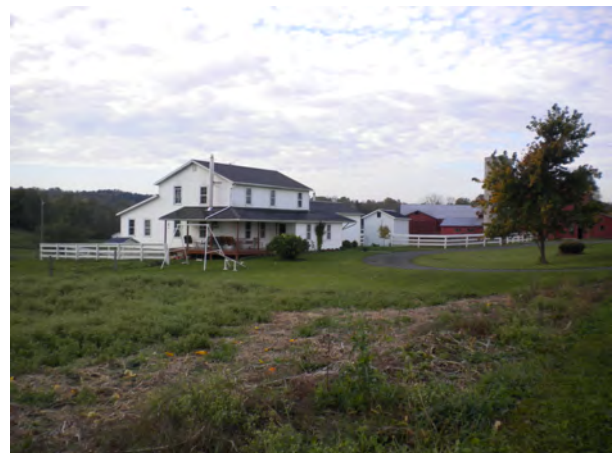
House, facing SW
