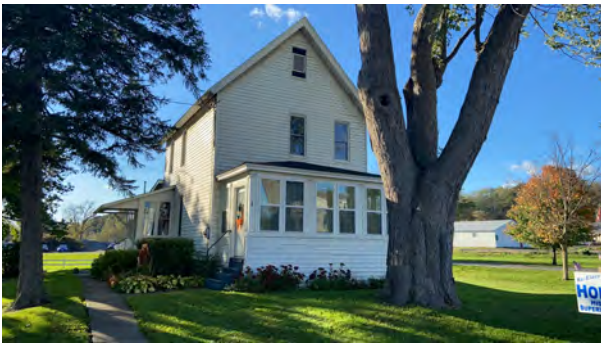
Facade (east elevation) and south elevation
