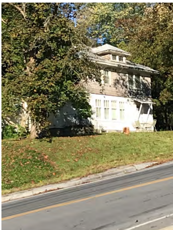
Facade, facing NW
