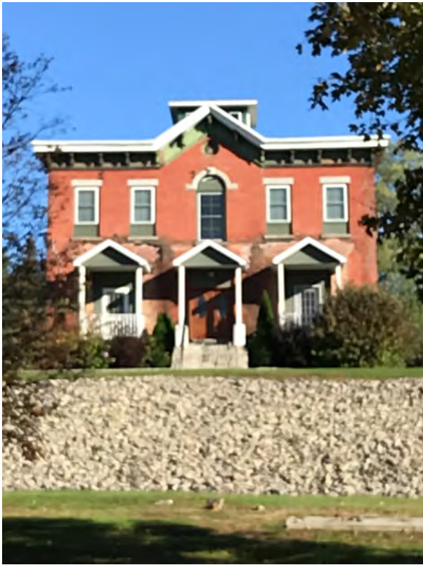
Facade, facing N
