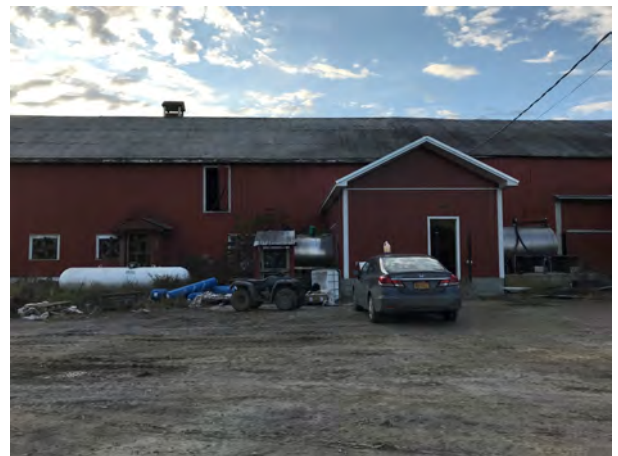
Ground Barn, facing W
