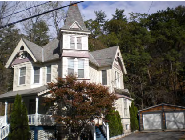
House, facing NE
