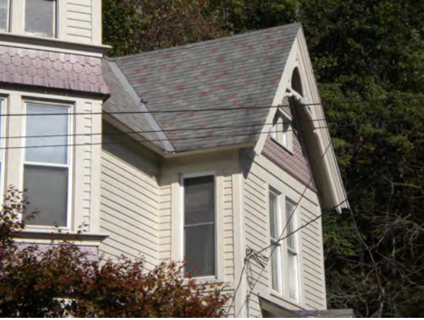
House, gable detail, decorative truss work in apex of gable
