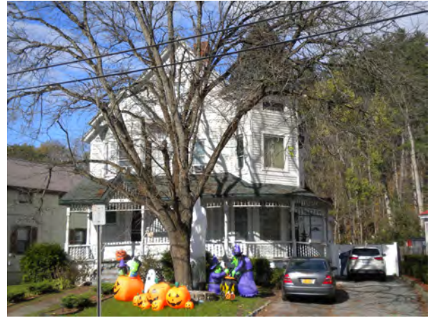
House facade, facing N
