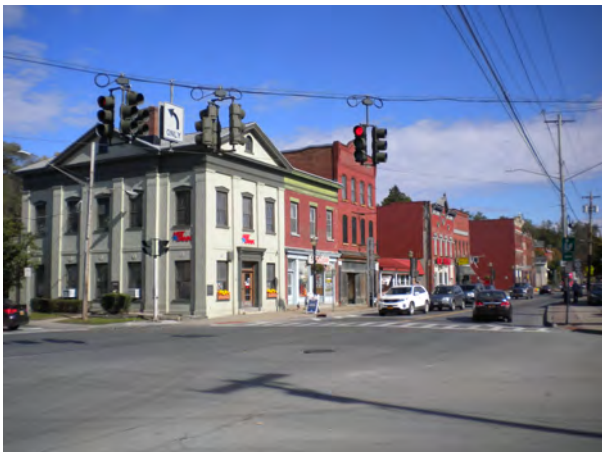
Bank, facing NE
