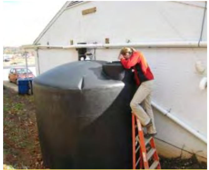
Figure 2.3.3 Inspecting the Storage Tank
