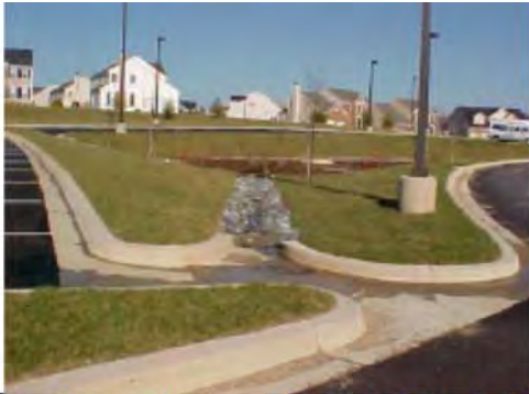
Curb cut – flow enters through defined place in curb
