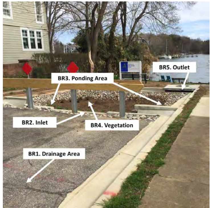
Figure 2.7.1. Key Areas for Level 1 Inspection of Bioretention
