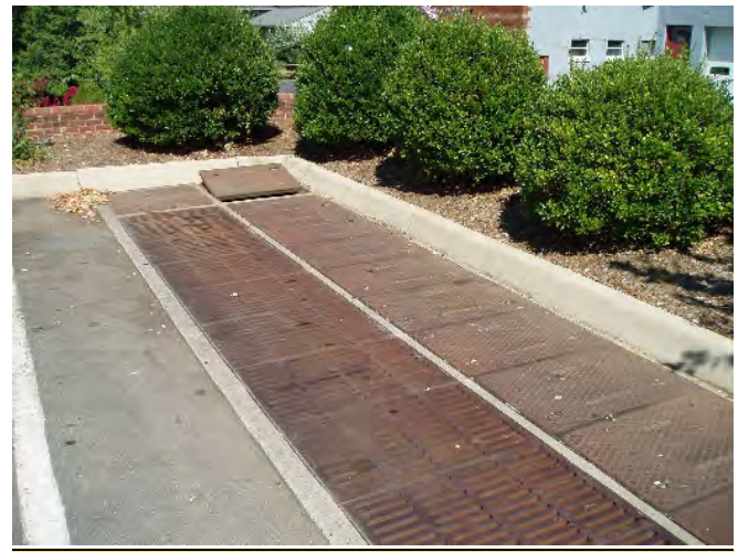
Figure 2.12.3. Key Areas for Level 1 Inspection of Sand and Organic Filters
