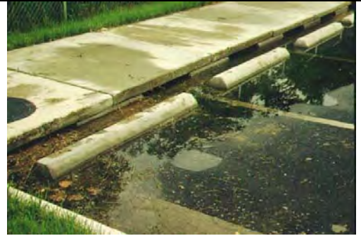
Standing water on the parking lot is evidence that this perimeter sand filter (under the sidewalk) is clogged.
