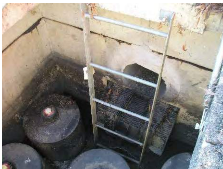
Figure 2.12.2. Examples of underground filters: Left –Perimeter sand filter in a concrete box (photo shows the filter with the grate top off as the filter is being maintained). The right-hand side is a sedimentation chamber filled with water and the left-hand side is the sand filter chamber. Right –Underground vault filter with special organic filter media inside cartridges.
